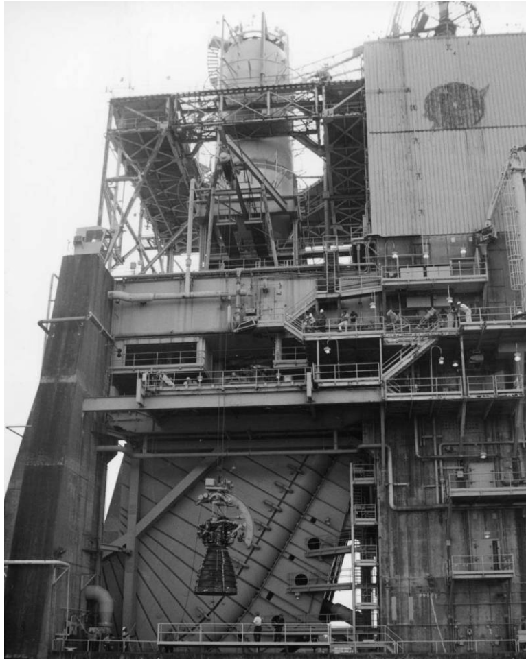
Figure C-5. A SSME being lifted into Stand A-2 at SSC for testing, camera facing east, 1996. Source: John C. Stennis Space Center, SIRS, 96-427-13, accessed at http://www.ssc.nasa.gov/sirs/scripts/xmlWelcome.pl .
